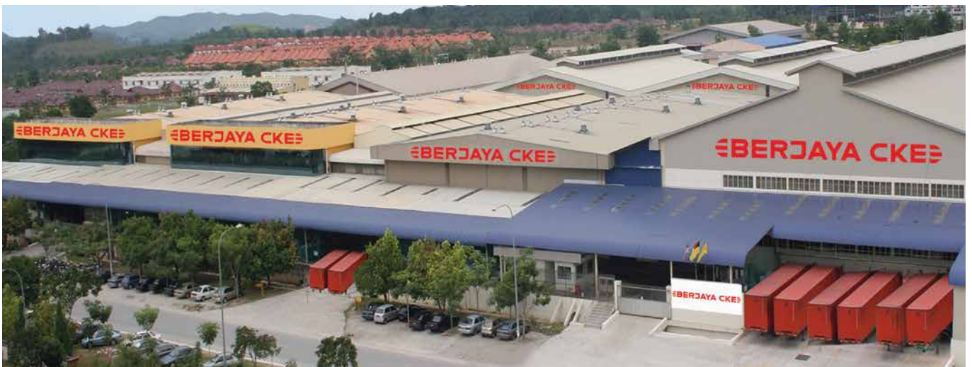
Manufacturing Plant In Negeri Sembilan, Malaysia
