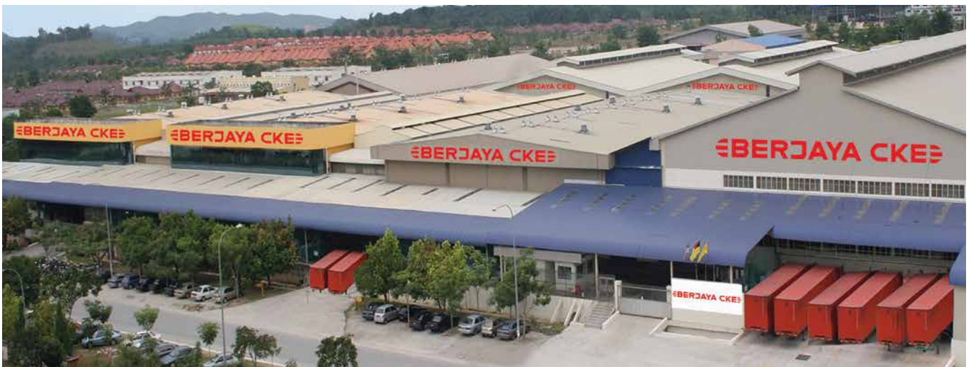
Manufacturing Plant In Negeri Sembilan, Malaysia
