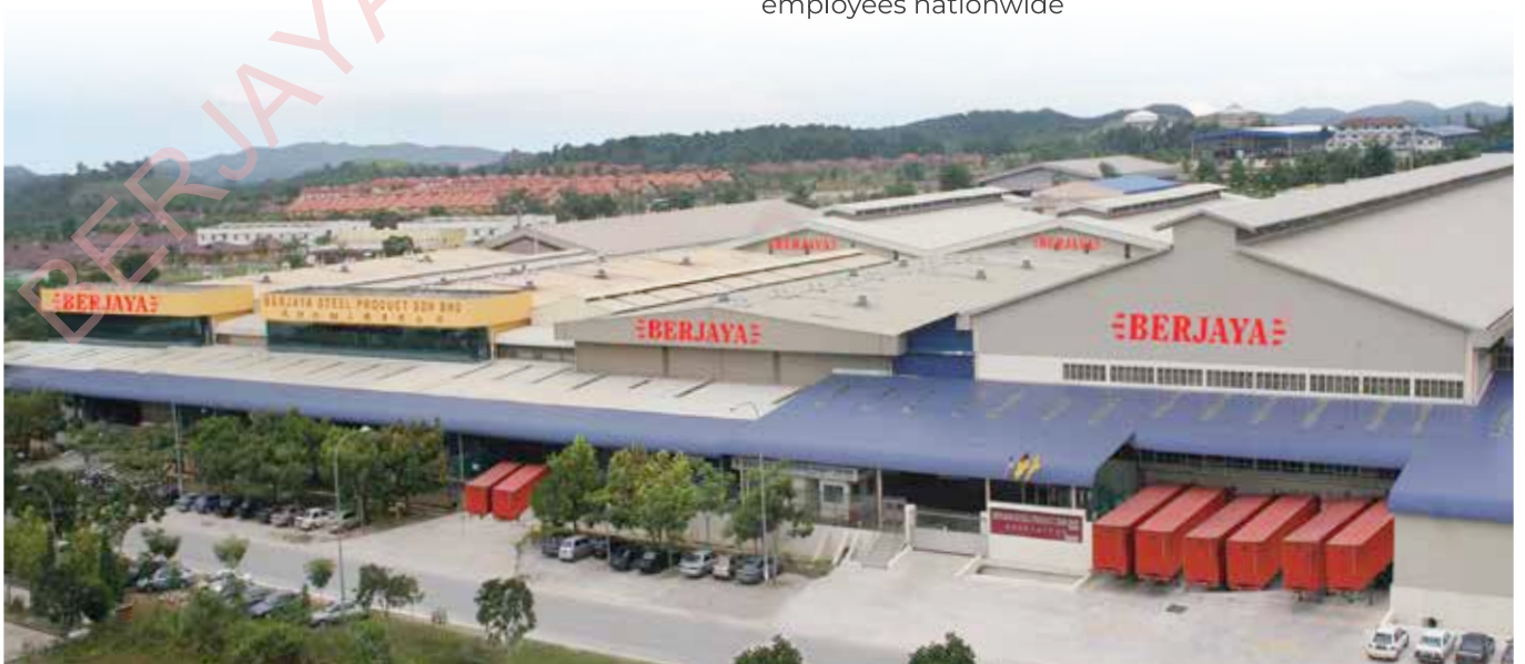
Manufacturing Plant In Negeri Sembilan, Malaysia
